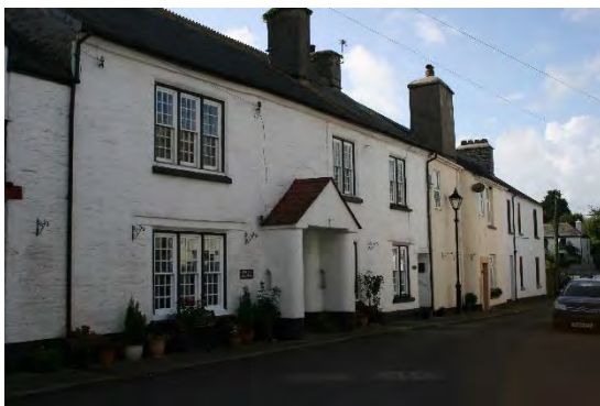
Figure 3.5 - High quality building design abounds in Landrake village and surrounding parish.
