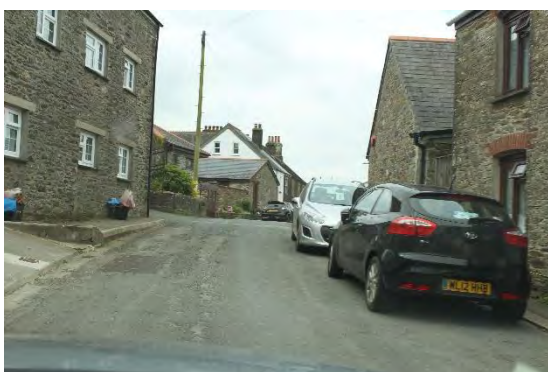
Figure 3.3- Buildings within the Parish historically were constructed from local materials and were of simple design
