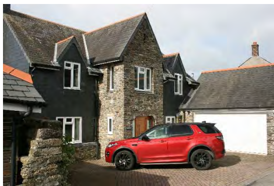
Figure 3.13 – This new dwelling has accommodated in-curtilage parking in a compatible manner. Parking should ideally be provided between houses and well back from the street, however this is not always possible.
