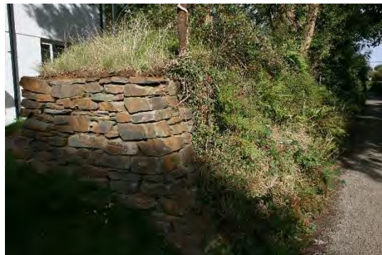
Figure 3.11 - Some recent developments in the Parish have made laudable attempts to complement traditional stone wall hedging techniques. Great care should be taken to chose stone that fits in with the local area
