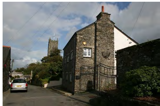
Figure 1.5 – An example of the variation of traditional building styles in the main village. This property fronting onto and responding to the tight street pattern running through the central historic core.
