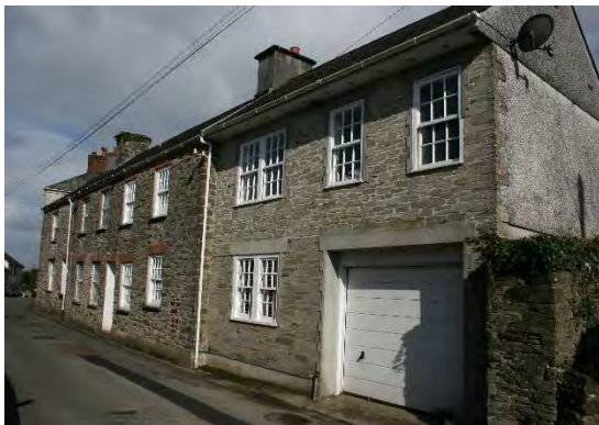
Figure 1.3 new build development that respects the neighboring buildings in terms of form and general detailing. However, the stonework is lighter in colour and has an uncharacteristic smooth finish. The garage door is out of kilter with the appearance of the street scene and that of the new dwelling which has been well executed.
